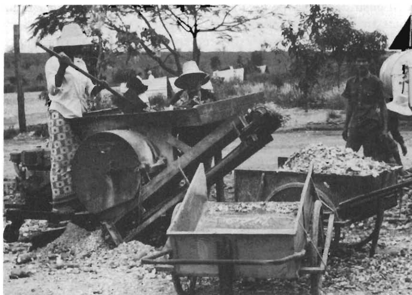
With cassava chippers and concrete drying floors, dried cassava can be produced at low cost. (Source: CIAT)
