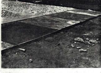
Figure 2. In 1984 the associations are increasing their drying capacity by 125%, allowing them to produce 2000 t of dried cassava per year. Using iron reinforcing bars and expansion spaces between concrete slabs, as recommended by CIAT, farmers make their own enlargements.
