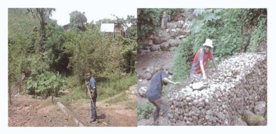
Figure 28. La Pimienta wetland, Yorito, Honduras (Left photo). Building the wetland stone wall (Right photo).
