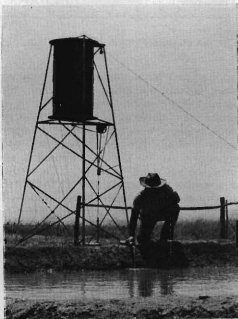
Carimagua windmill mounted on 5.5 meter galvanized steel tower. Reservoir in foreground is formed using soil from well excavation
