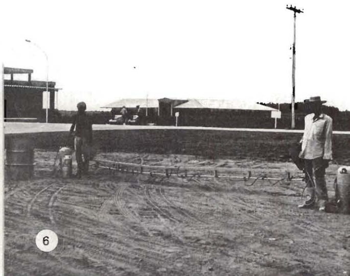
Back pack sprayers and 6 meters boom built in CIAT shops.
