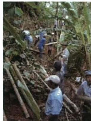
Figure 6. Constructing sediment barriers for erosion control.
