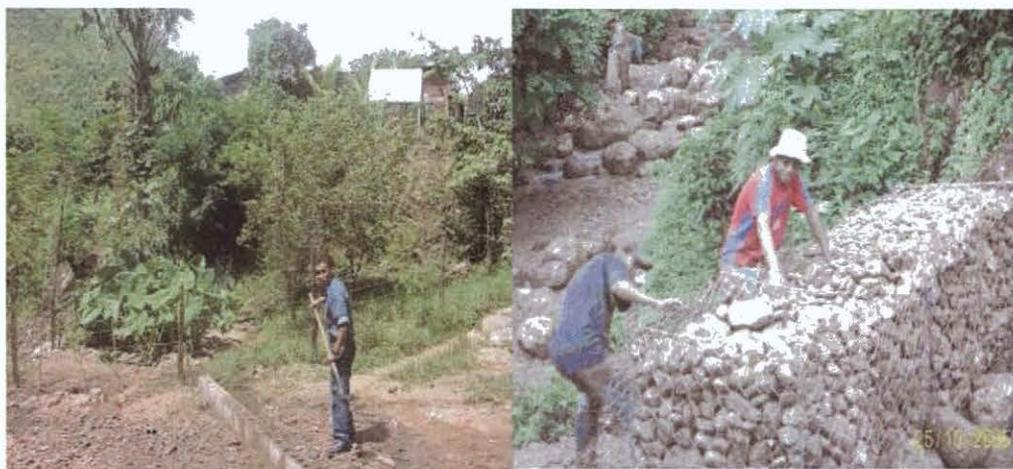
**Figure 28.** La Pimienta wetland, Yorito, Honduras (Left photo). Building the wetland stone wall (Right photo).
