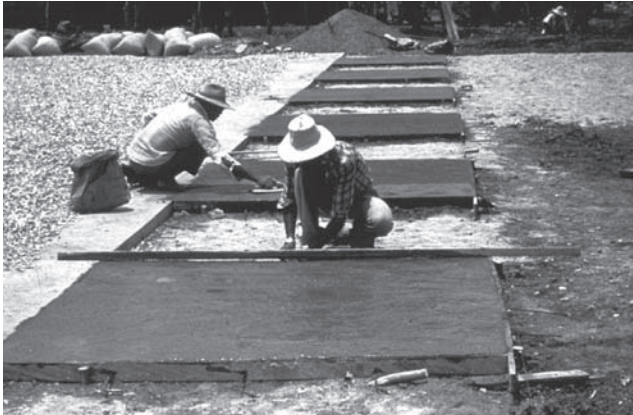
Figure 21-15. Expansion joints are placed between concrete slabs (A), together with iron rods (B).
