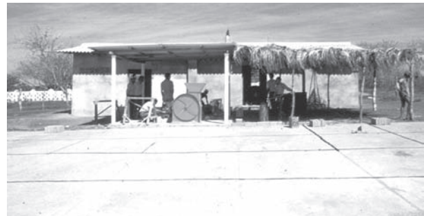
Figure 21-17. View of the roofing complex used to cover the cassava chipping machine and to protect the fresh cassava roots received for processing.
