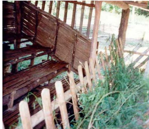
Photographs 7 and 8. The innovative goat house in Lumbia: the stair-like or tribune construction of the half open floor allowed for easy dung collection.
