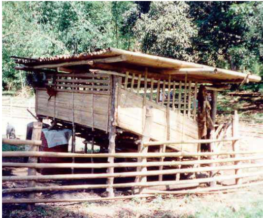
Photographs 7 and 8. The innovative goat house in Lumbia: the stair-like or tribune construction of the half open floor allowed for easy dung collection.
