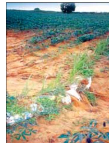
Photo 5. Repair of eroded gully using soil-filled bags and planting vetiver grass in the collected sediments
