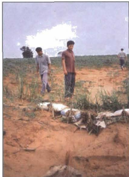
Photo 21. Soil bags anchored with sticks and placed across the gully trap soil allowing the replanting of vetiver grass in the sediments.
